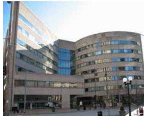
6 N. MAIN STREET BUILDING
