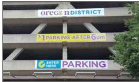
OREGON DISTRICT PARKING GARAGE
