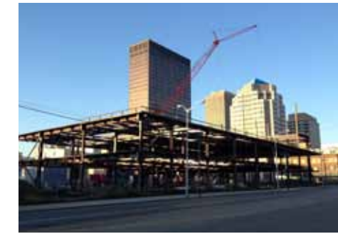
NEW CARESOURCE OFFICE TOWER CONSTRUCTION
