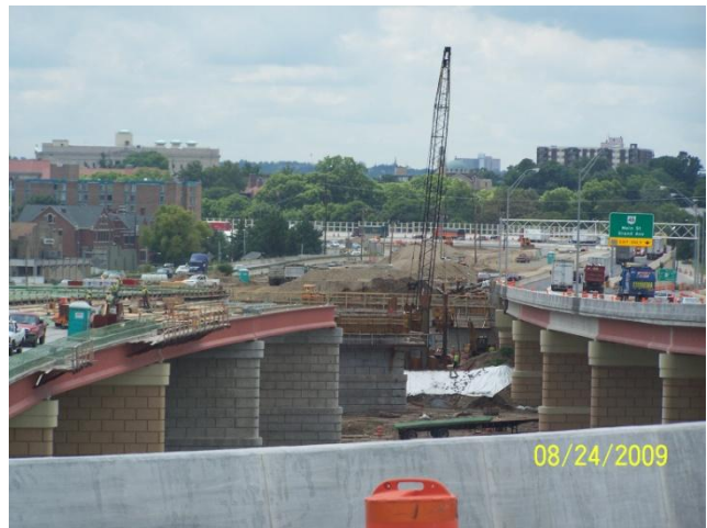
Looking south across the river bridges currently under construction.
