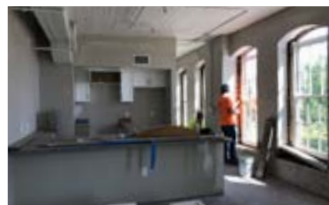
CONSTRUCTION ON THE WHEELHOUSE PROJECT
